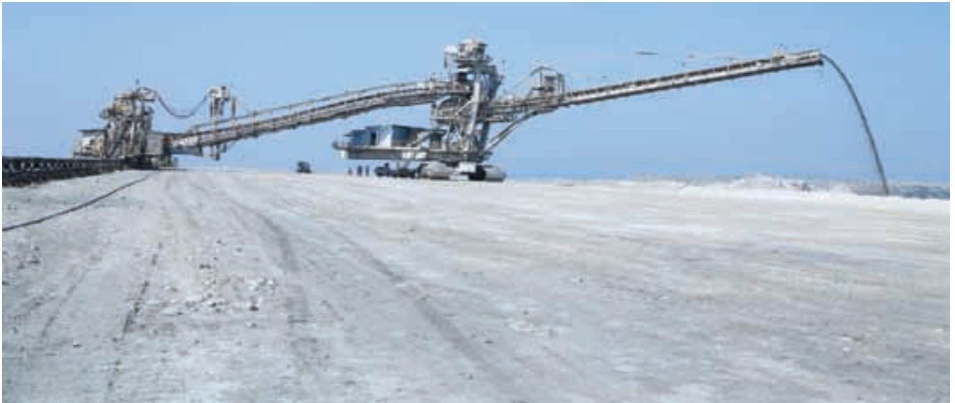
Spreader of the Input Crusher and Conveyor in RG OC-2 (RG-3 Area)
